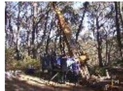
Goldstar drilling at its Walhalla gold project in Victoria.
